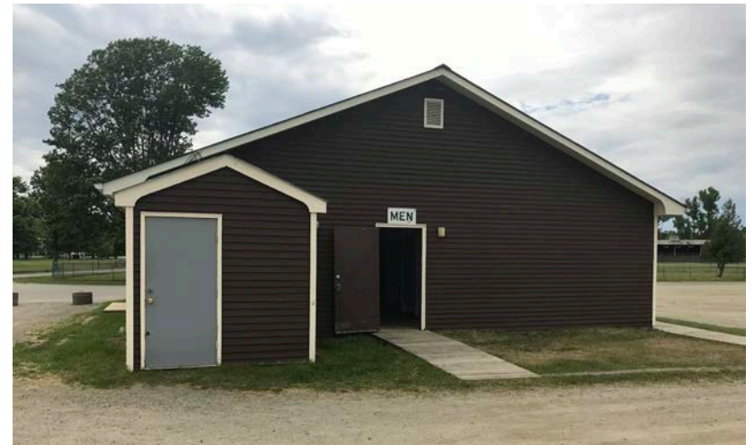
Gardner Memorial Park staff offices and bathroom facilities
